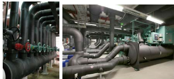
Fig. 1 Use of elastomeric foam insulation (FEF) in pipe insulation
