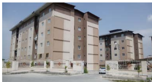
Fig. 1 A picture of the residential complex of Talashgaran
