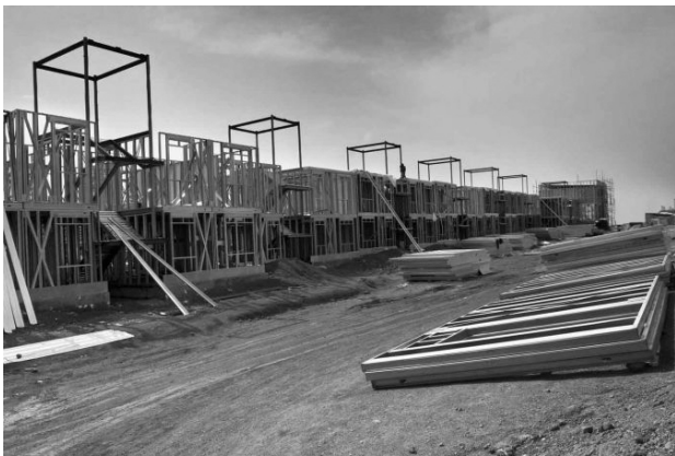
Fig. 1 Steel Staircases in LSF
